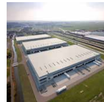
SMARTLOG DEN HAAG HARNASKADE YEAR OF CONSTRUCTION: 2018 81,251 M 2
