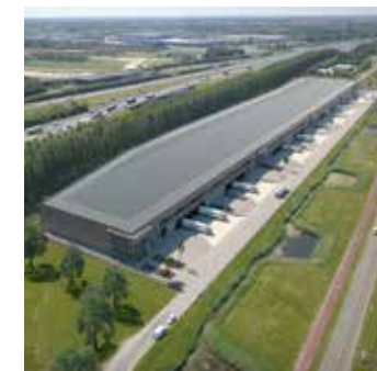
SMARTLOG RIDDERKERK SCHAAPHERDERWEG YEAR OF CONSTRUCTION: 2018 49,700 M 2
